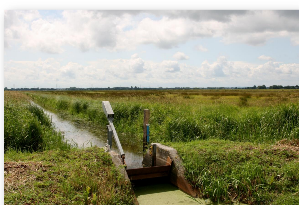
FIG 7: Ditch management by adjustable weirs.
